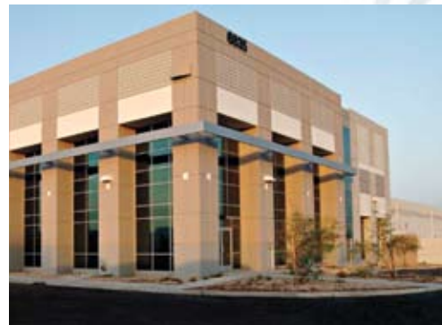
The Buckeye Logistics Center is another Alter Group project.
